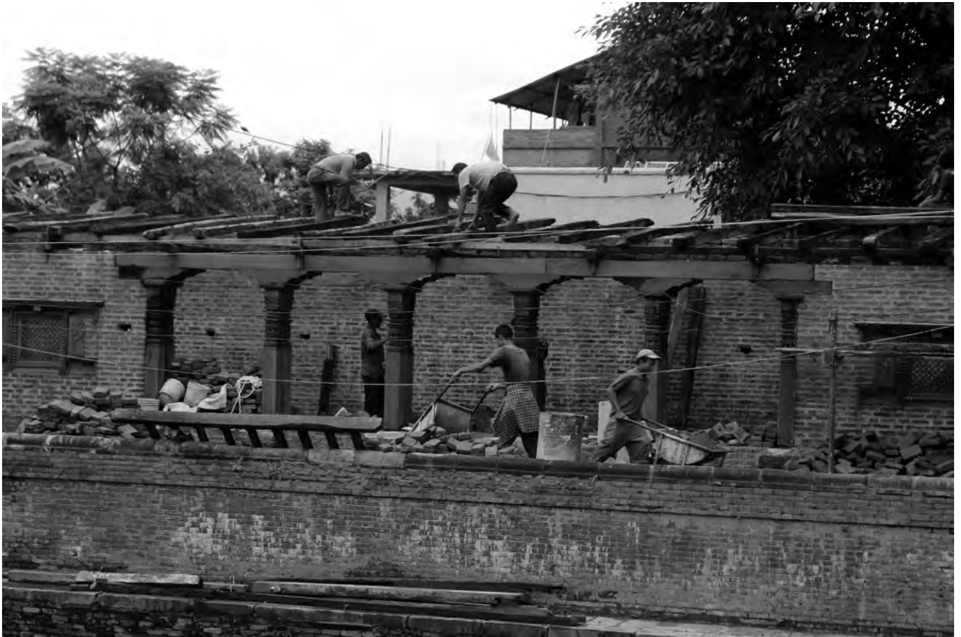
Photo 1: Tawa Sattal is being reconstructed under contractor-led reconstruction. Photo: Sara Shneiderman.
