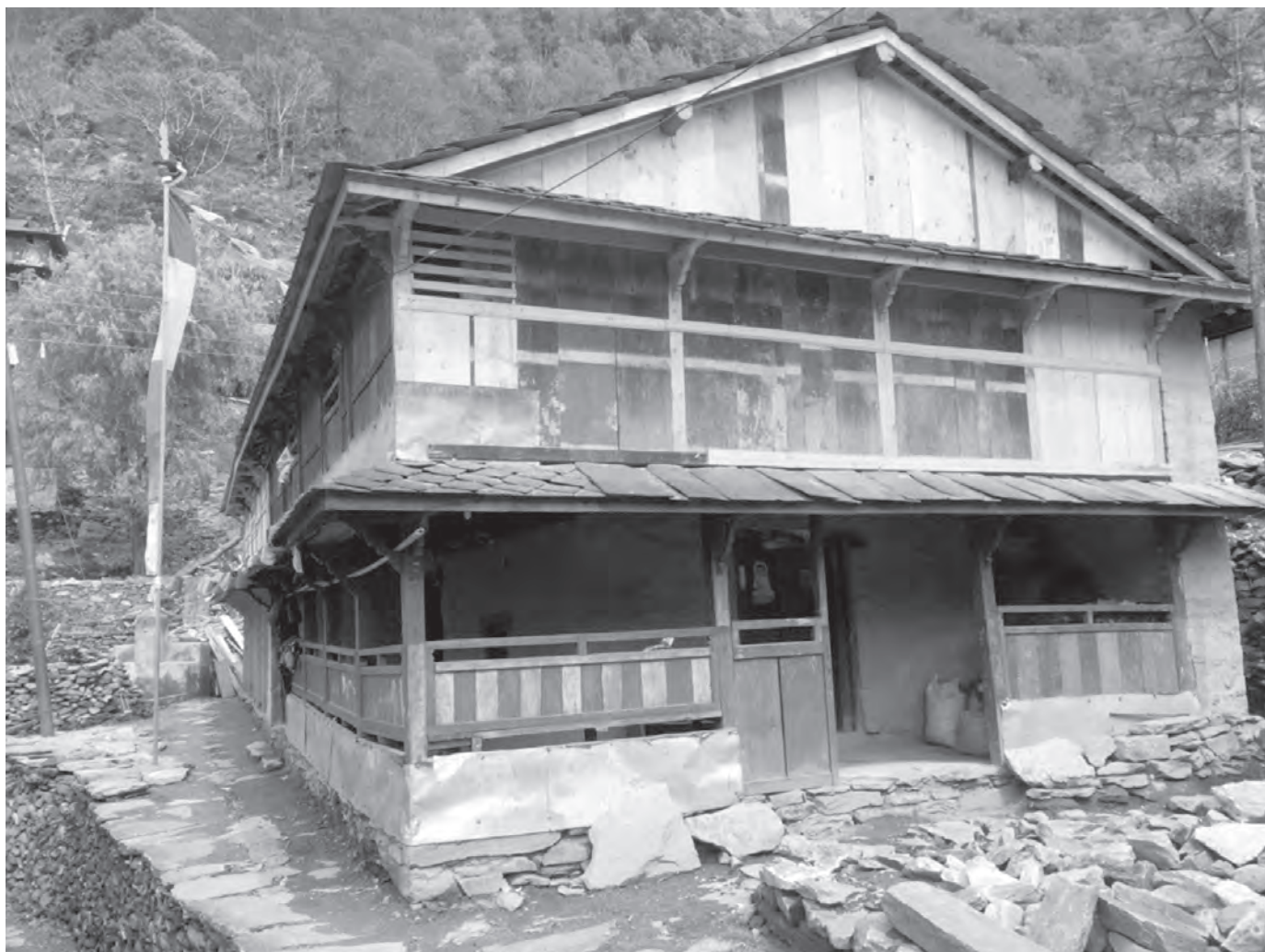
A earthquake-damaged house in Borang, Dhading, previously made of stones, then repaired by building the first floor and the attic with wood and roofing it with CGI sheets. Photo: Bina Limbu
