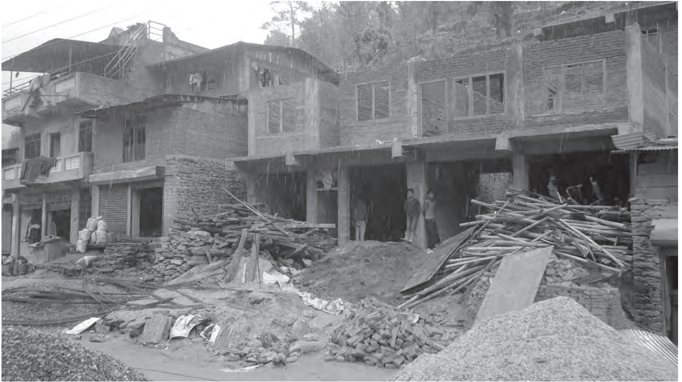
New construction in Kartike Bazaar, Sindhupalchowk. An RC frame house stands next to a load-bearing house that has used stones on the ground floor and bricks on the first. Photo: Manoj Suji.
