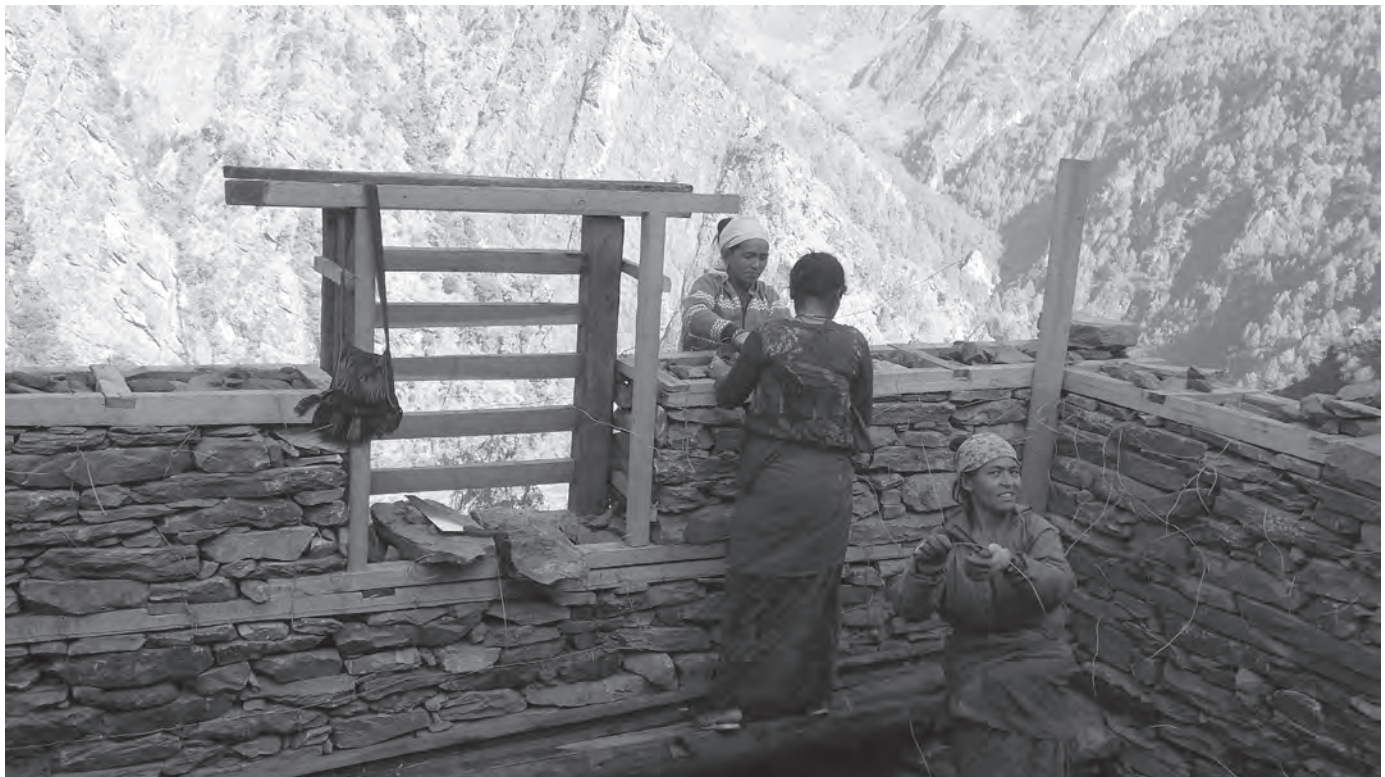
Women masons in Borang undergoing training to build earthquake-resistant houses. Photo: Manoj Suji
